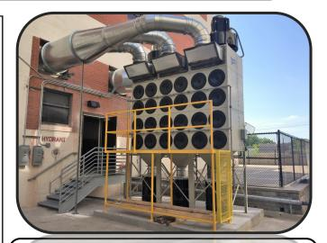
RP8-3 with Top Mount Fans & Intelli-Touch Controls, Ducted to Source Capture Arms in an Iowa Vo-Tech School
