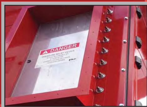
NFPA/OSHA compliant explosion vent.
