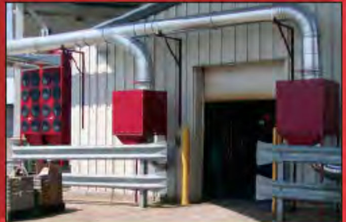
RPB-2 with spark arrestors collects laser smoke.
