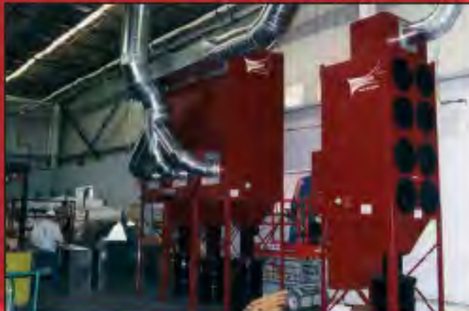
RPB-3 and RPB collect silica/carbon impregnated NEUSTRON DUST.
