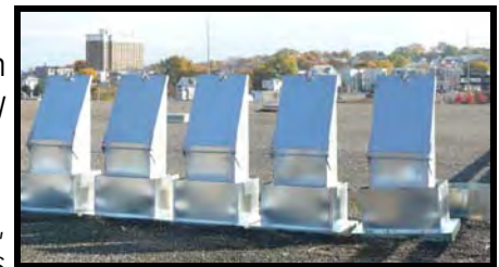
Roof Penetrations for Explos. Vents
