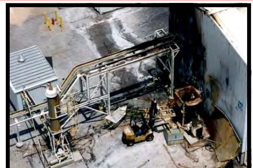
Conveyor Fire caused secondary explosion in this manufacturing facility.
